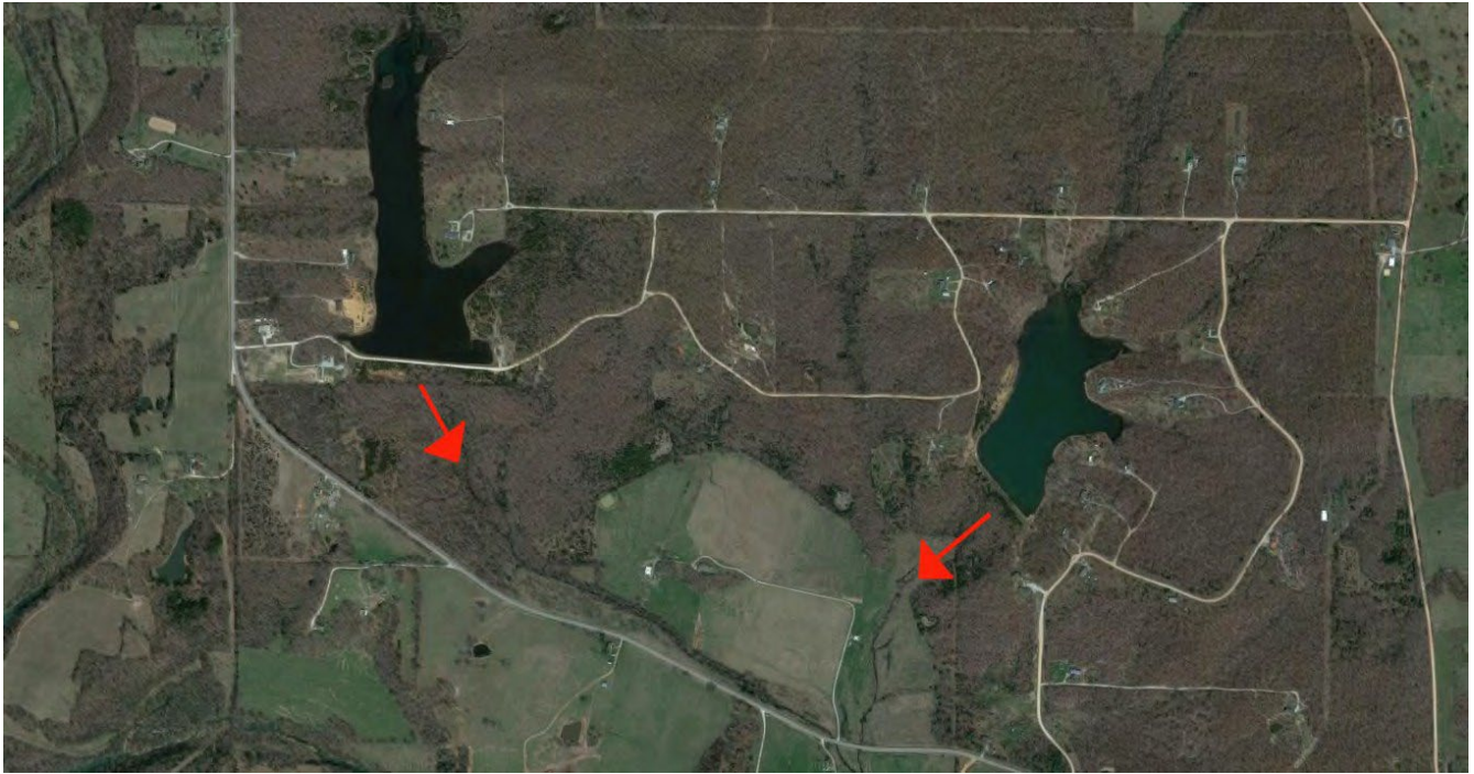
Figure 3.14. Stace Shannon (left) and Brent Lake (right) Dams
