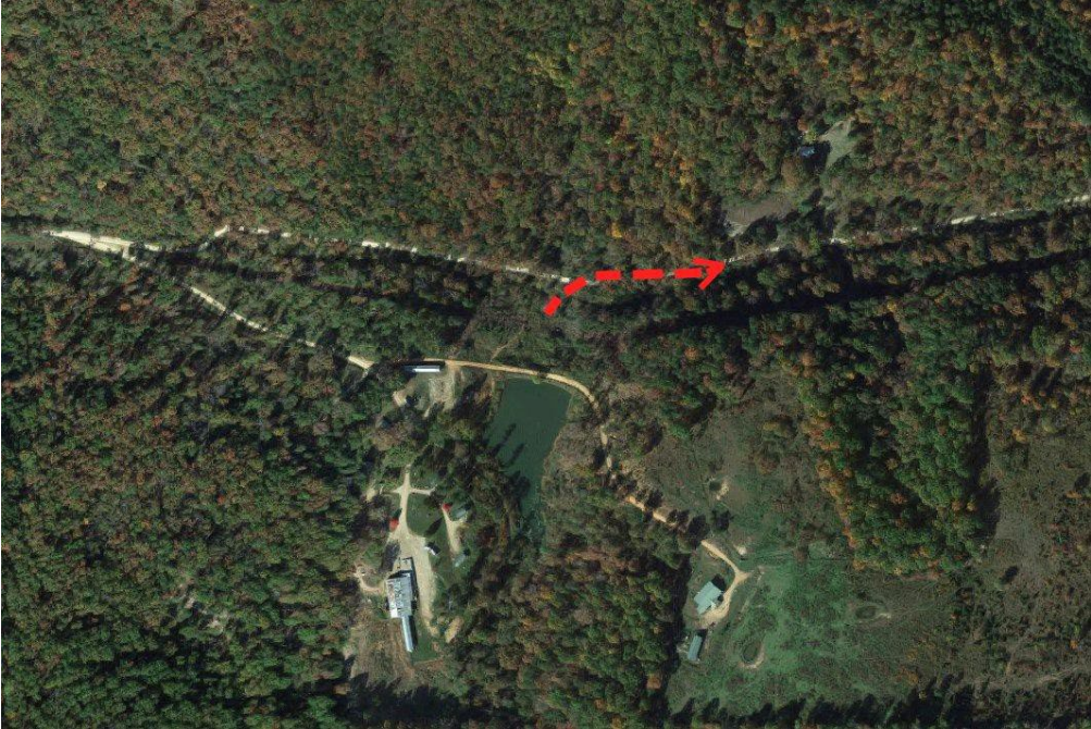
Figure 3.8. Coldwater Ranch Dam
